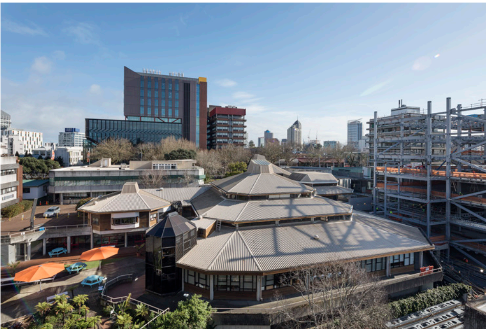
Fig. 1 The complex roof forms, with the Architecture and Planning Library in the foreground. It sits back-to-back with the Design Theatre (under the turret), with the Dean's Office to its left (south), and the Conference Centre Lecture Theatre and so-called Flat Floor Space to the right (north). Construction of a new building for the Faculty of Engineering is underway.
