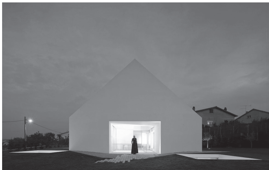
Leiria House Renders and Section, Leiria, Portugal 2008-2010. [Courtesy of Aires Mateus e Associados & Francisco Aires Mateus Arquitectos, with photography by FG+SG - Fernando Guerra, Sergio Guerra]
