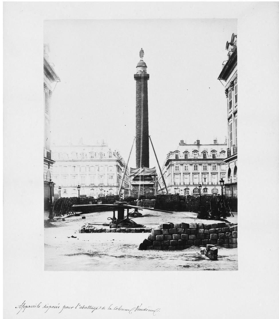
Fig. 2 Bruno Braquehaïs (1871). The Vendôme Column rigged for demolition. Plate from album "Siege de Paris, 1870-1871". [Photograph, Collection Centre Canadien d'Architecture/Canadian Centre for Architecture, Montréal]
