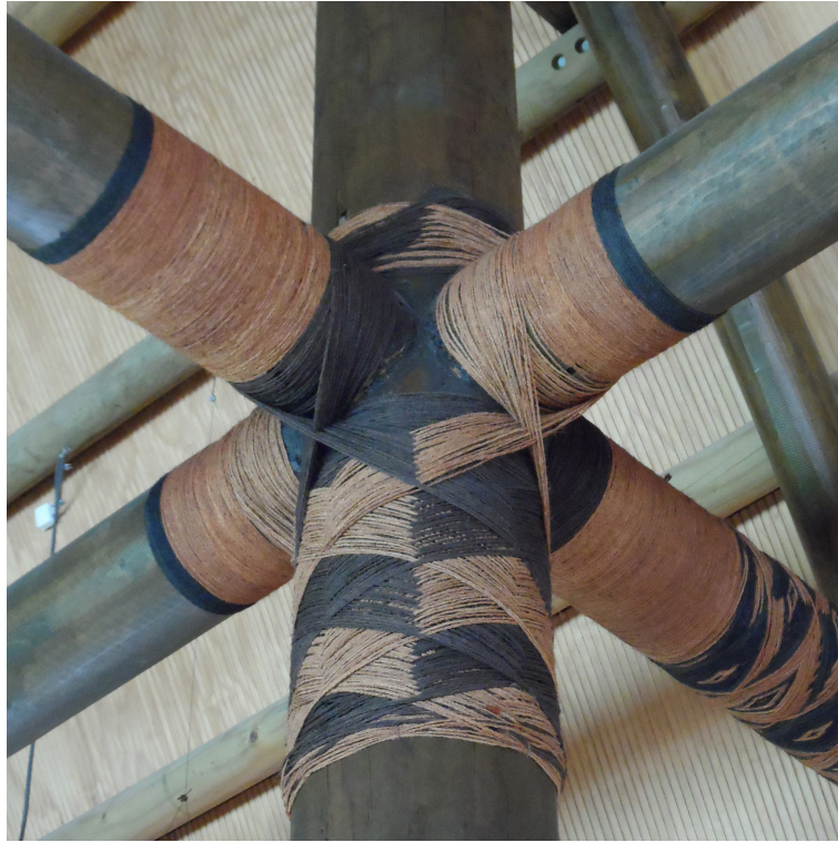
Fig. 4 Lalava covering post/beam connection [Photo: author, 2017]
