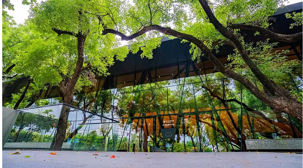
Fig. 6 Main entrance with V-shaped steel structure [Photograph: Pan Mengan, 2020]
