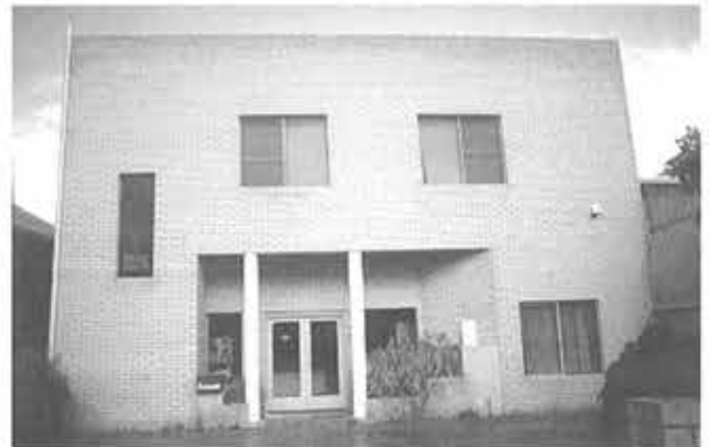
Office warehouse, East Perth.
