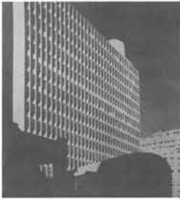
OSCAR NIEMEYER. Ministry of Education. M.M.M. ROBERTO. A.B.I. Building in Rio de Janeiro.
