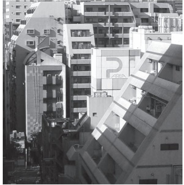
Typical bevelled building forms in Japan (photo by Tom Daniell).
