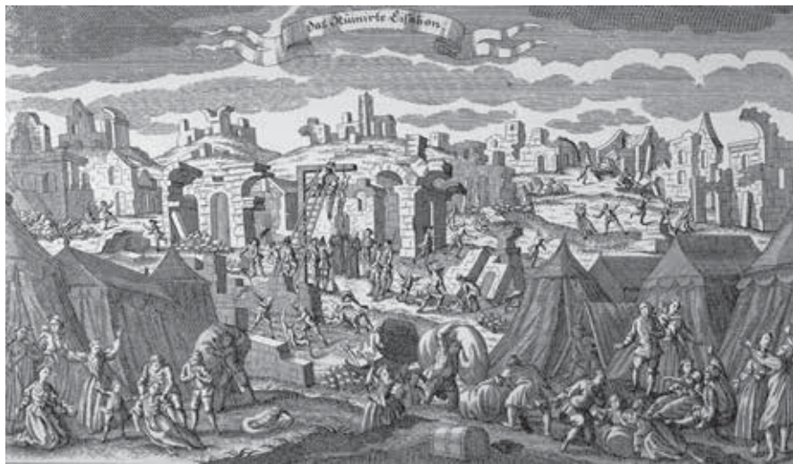
Fig. 1 The Ruins of Lisbon (1755) German copperplate engraving, artist unknown. [Source: National Information Service of Earthquake Engineering (NISEE), University of California, Berkeley]
