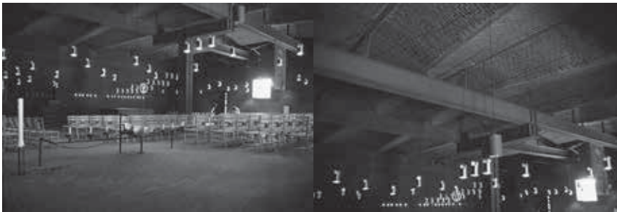
St Peter. Main chapel, brick floor, steel framing and brick vaults.
