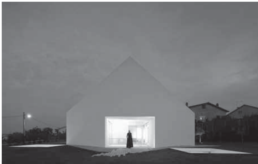
Leiria House Renders and Section, Leiria, Portugal 2008-2010. [Courtesy of Aires Mateus e Associates & Francisco Aires Mateus Arquitectos, with photography by FG+SG – Fernando Guerra, Sergio Guerra]
