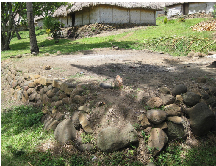
Fig. 7 A vacant yavu in Navala Village, emphasising the intentional permanence of this bure feature, clearly more so than its roof and walls [Photograph: Charmaine 'Ilaiū Talei, 2010]
