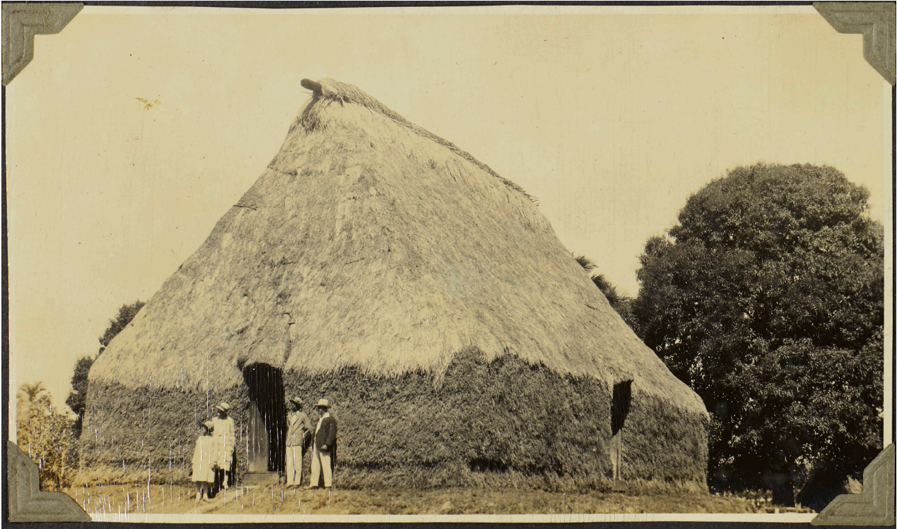
Fig. 1 Chief Josese Nabuta's house at Ba, Fiji (1928) [Photograph: Milton Vickery, Auckland Libraries Heritage Collections 1467-ALB274-122-3]
