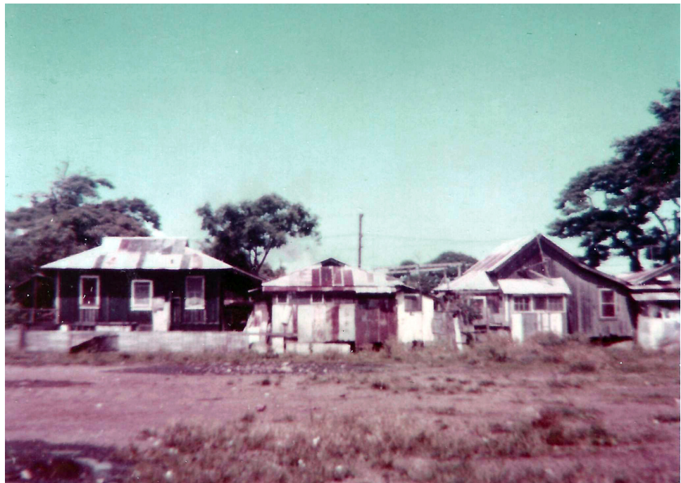
Fig. 6 The 'camp' on Robelo Lane in Kapalama, Honolulu, before being torn down [Photograph: Hampton Miller, ca. 1960]
