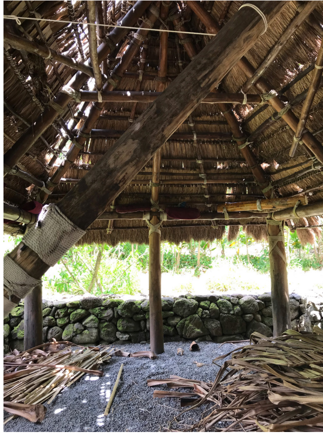
Fig. 3 The interior of a hale pili at Ho'oulu 'Āina [Photograph: James Miller, 2019]
