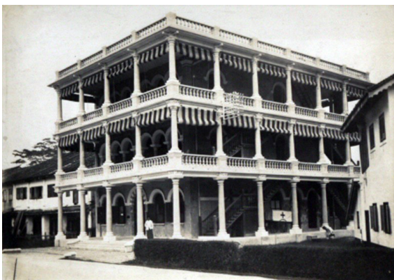
Fig. 3 Top: The European Hospital and Dispensary was built in 1909 and was the first public building in Sarawak to be over two storeys high. It had a concrete frame supported by bakau (mangrove timber) piling. Bottom: The main entrance to Sarawak General Hospital in 1930 [Photographs: National Archives United Kingdom]
